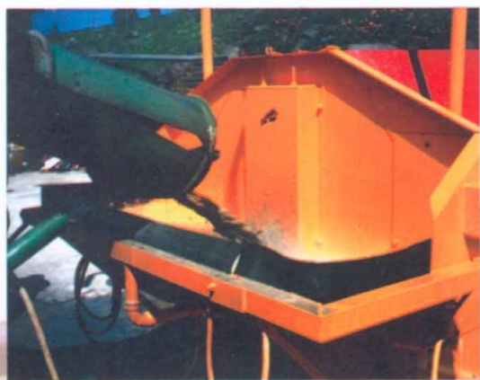
The concrete is discharged from the truck mixer into the feed tray.
