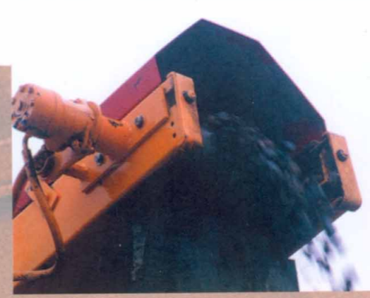
The aggregate is removed using a conveyor.
